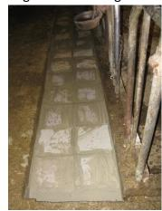
the manger made it plenty wet. We trowled the concrete mix in and laid the tile imbedded in the mix. We used a level to try and keep the pitch to one direction and keep our new surface tiles somewhat level. 12"x 12" tiles cost \$.50 per tile at
